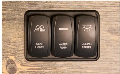
Figure 5-15. Switch Control Panel located on upper cabinetry
