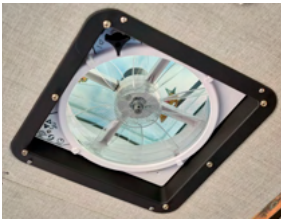
Figure 3-2. Fan (interior view)
