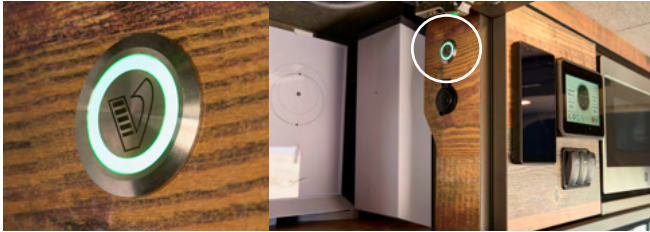
Figure 2-1. ON/OFF Pushbutton and its location in the upper Connectivity Cabinet
