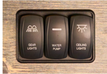
Figure 4-1. Upper Cabinet Switch Control Panel
