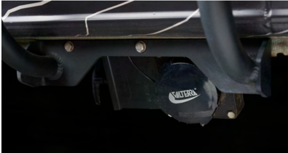
Figure 4-5. Grey Water Tank Drain
